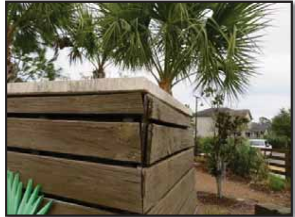
Figure 4 – Warped Boards.
